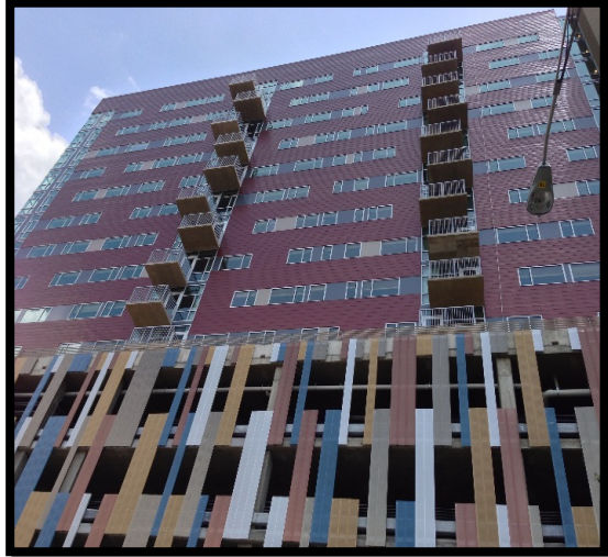
A student housing building at the University of Texas at Austin, where anodized aluminum was used to make shingles that are incorporated into the façade design. Perforated anodized aluminum sheets on the building's garage also help the building to meet ventilation requirements while coordinating with the overall building design. Photo Credit: Lorin Industries, Inc.
