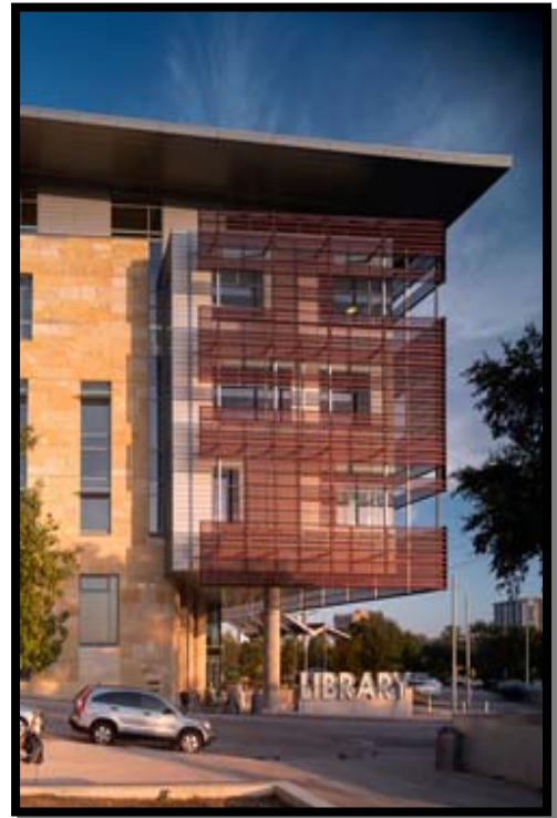
Perforated anodized aluminum is a central façade design element in the recently constructed central library in Austin, Texas. Photo credit: NicLehoux
